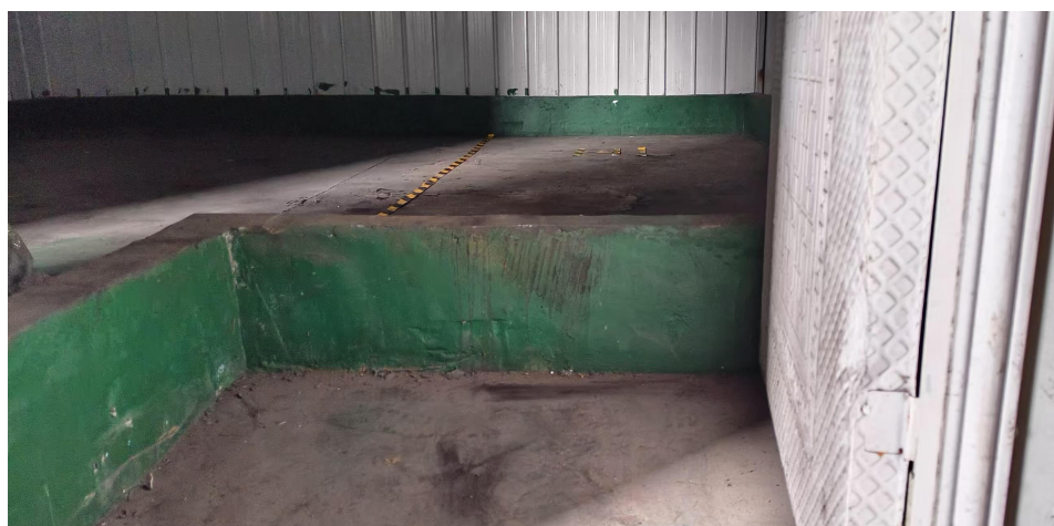
危废仓库门口围堰
